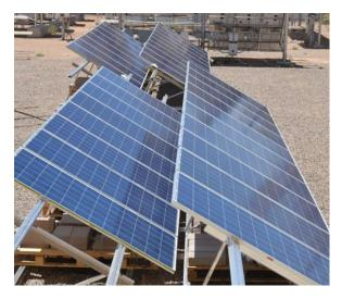
Figure 3.2.1 West-facing, portrait configuration of conventional solar panel and P-Series arrays
