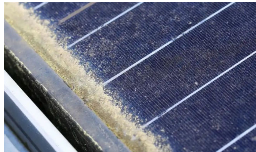
CRUD BUILDUP AT BOTTOM OF PANELS INSTALLED BELOW 10 DEGREES PITCH
